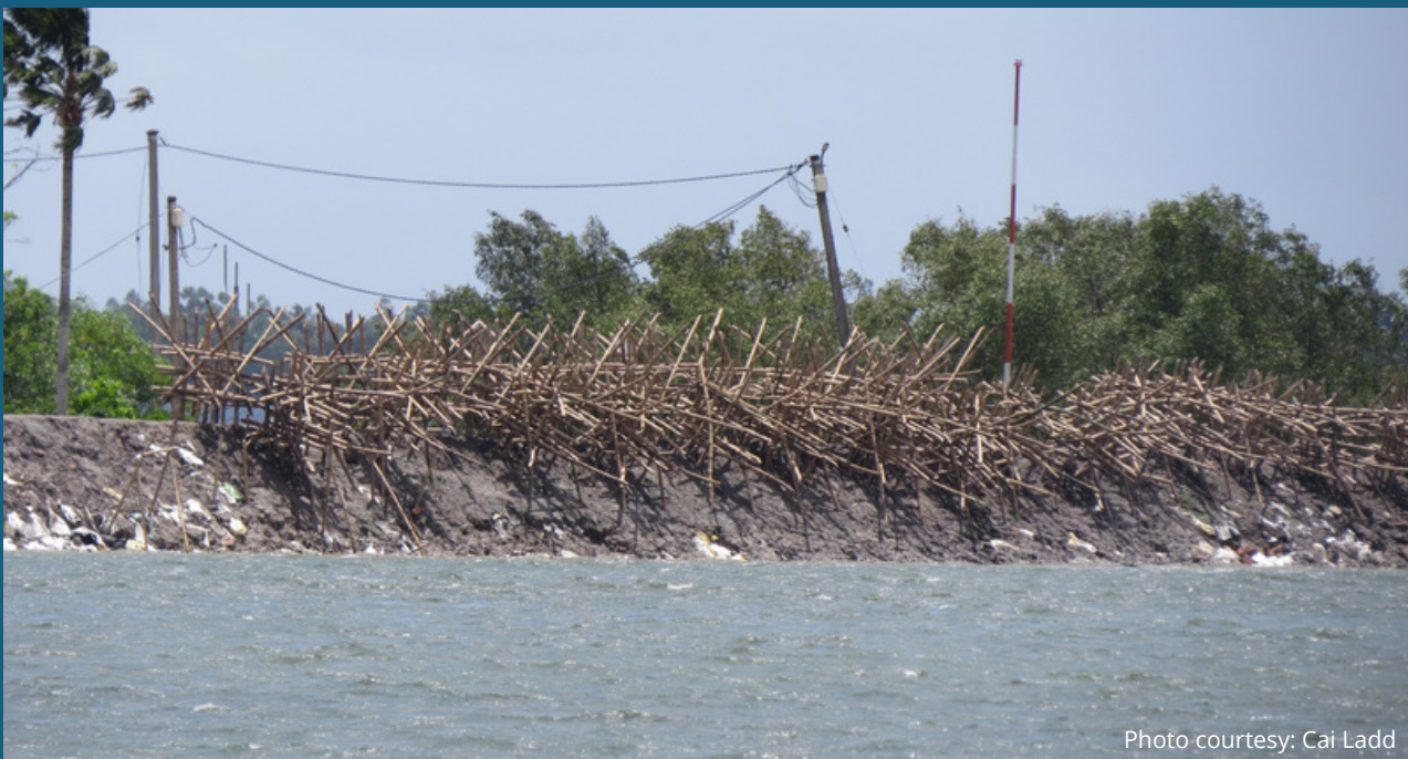
Porcupine System used to trap sediments and prevent erosion in Indian Sundarban
